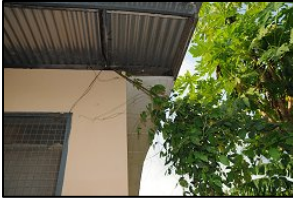
The cable leaves the rear of Father Oppong's room...
