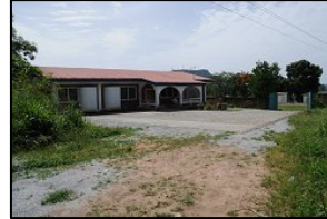
...under the block paved driveway...
