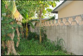
...over the wall and down into the ground...
